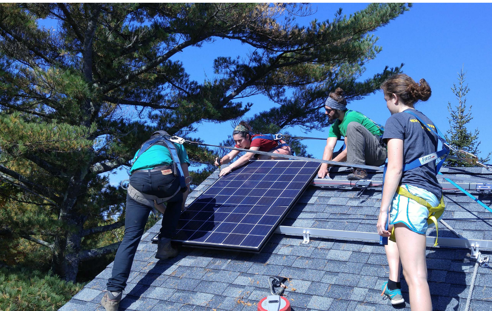
Bates College students install solar panels. Photo credit: Tom Twist.
