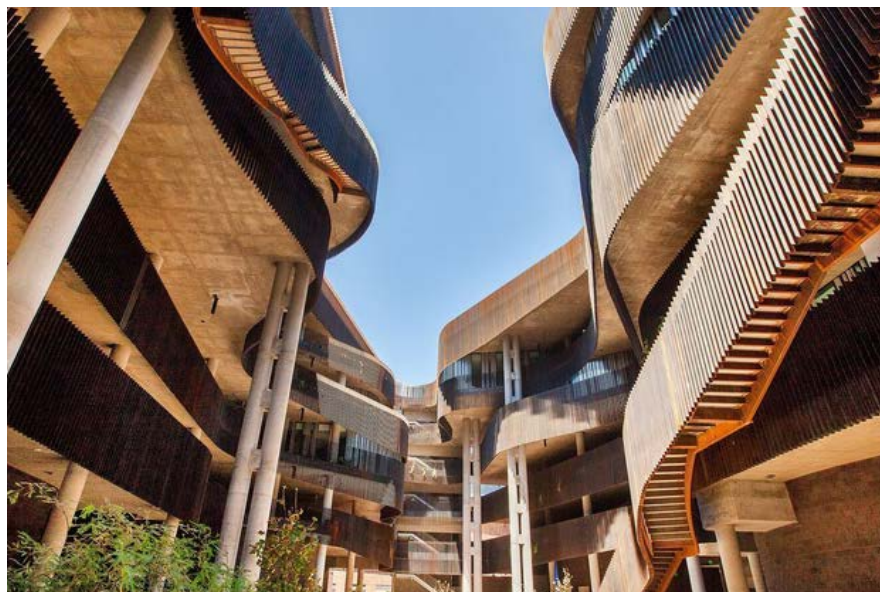
The ENR2 building at University of Arizona was formally dedicated on Sept. 10, 2015. Photo credit: John de Dios
