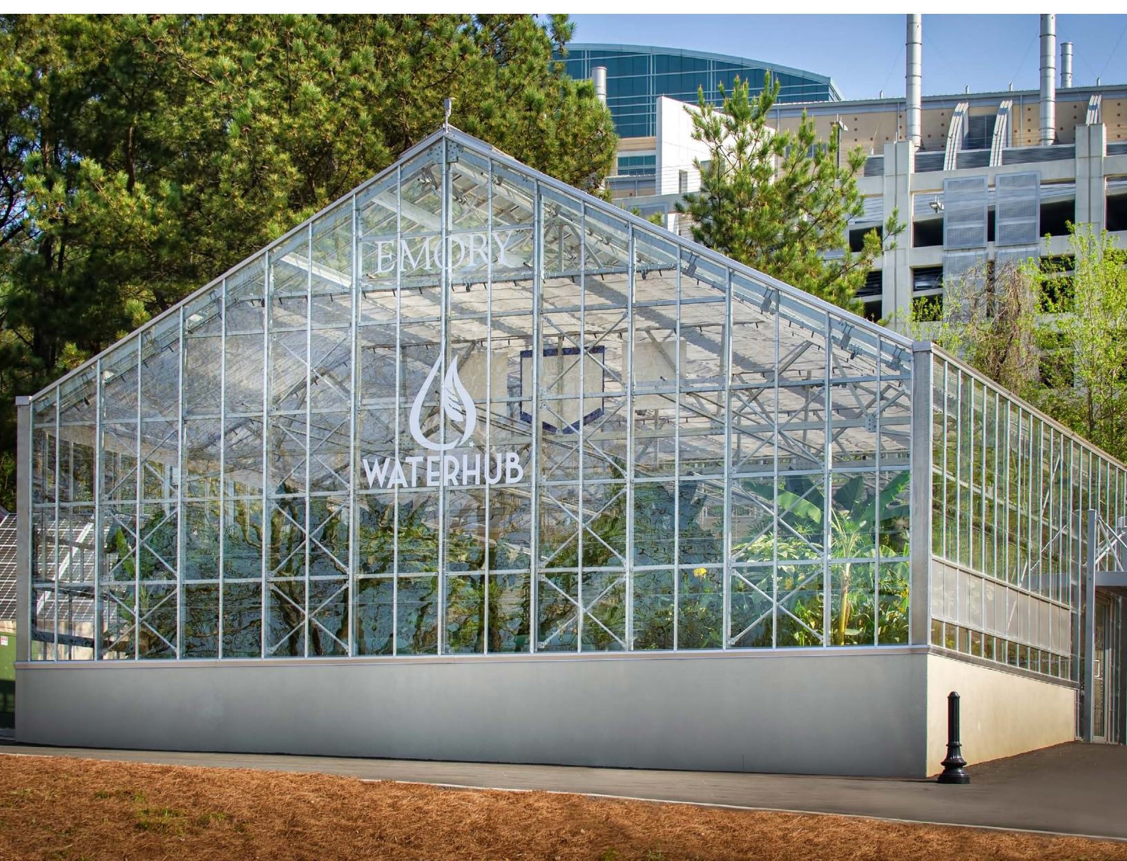
The Water Hub water reclamation and reuse system at Emory University. Photo credit: Sustainable Water
